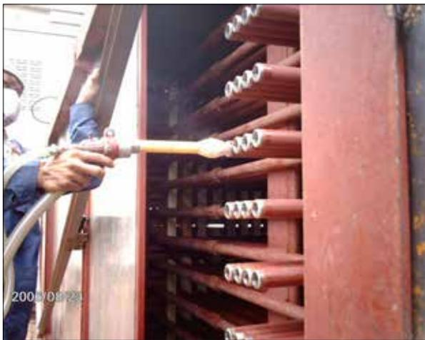
**VpCI®-309 Nitrite Free Powder** is a Vapor phase Corrosion Inhibitor powder for corrosion protection of ferrous metals in recessed areas, interior cavities, and voids. VpCI®-309 provides an extremely efficient dry method to protect metals within an enclosed space. The VpCI® vaporizes and adsorbs on all metal surfaces reaching all exposed areas including recessed sections and interior cavities. VpCI®-309 SF, a silica-free version, is available upon request.
